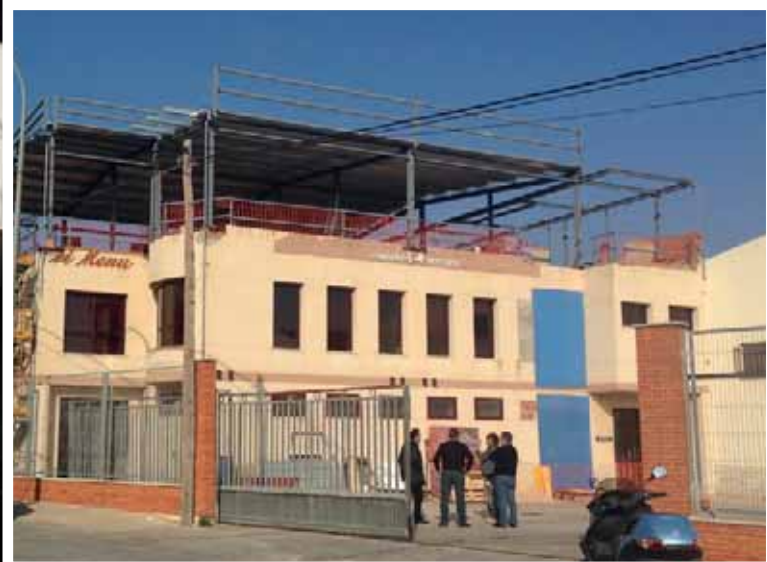
Offices building Castellón - Spain
