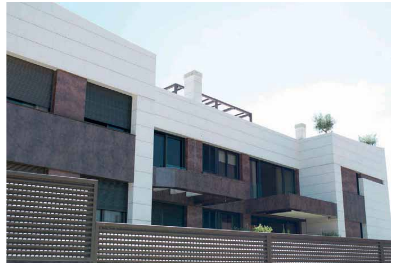
Residential building (MAdrid - Spain)
