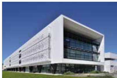
INSTITUT D' OPTIQUE D' AQUITAINE Location: Talence, France Studio: Cabinet d' architectes Nicolas Raguenau & Antonie Roux
