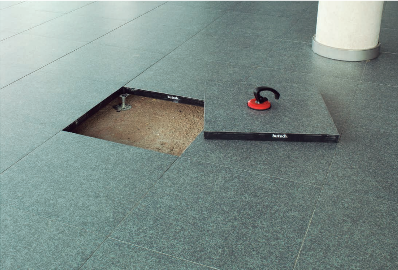
Technological building of UJI University (Castellón, Spain)
