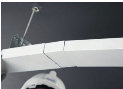
7. Join two profiles, leaving the joint piece at the profile ends.
