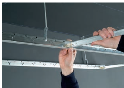
7. Install the 60 cm and 120 cm secondary profiles.
