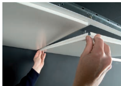
10. Exert pressure forward while we start raising the plate.
