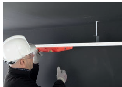
8. Check the trays resting on two profiles using the plate tabs.
