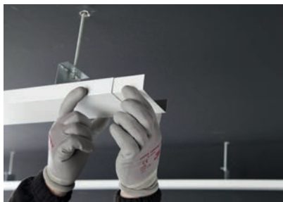
6. Install the joint piece at the profile ends.
