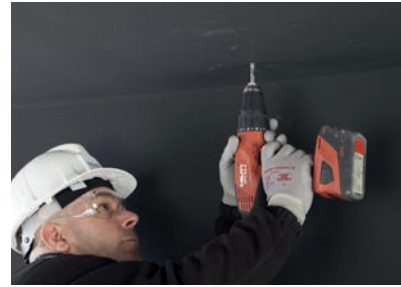
2. Mark the location of the hangings and make the holes.
