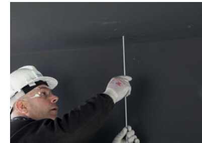
3. Install the stud and the threaded rod.
