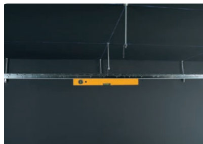
6. Check that the primary profiles are leveled.
