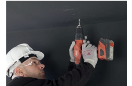
2. Mark the location of the hangings and make the holes.
