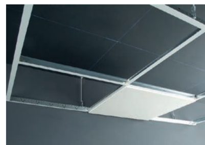
11. The plate will be fixed within the grid.
