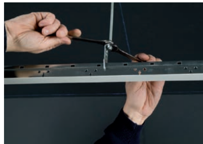
4. Join the primary profile with the rod using the nuts. (Use two nuts for each hanging piece)
