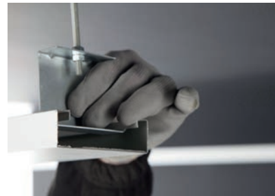
5. Join the hanging piece with the rod using the nuts. (Use two nuts for each hanging piece)
