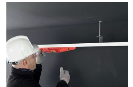
8. Check that the profiles are leveled.
