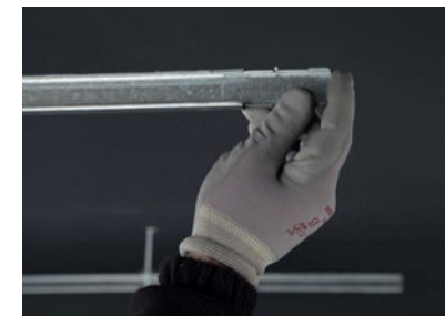
6. Install the joint load-bearing profile to join two load-bearing profiles, when necessary.
