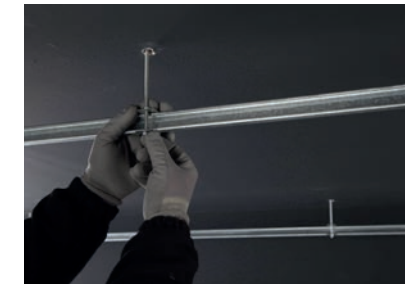
4. Install the clamping flange and the bearing profile.
