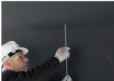
3. Install the stud and the threaded rod.
