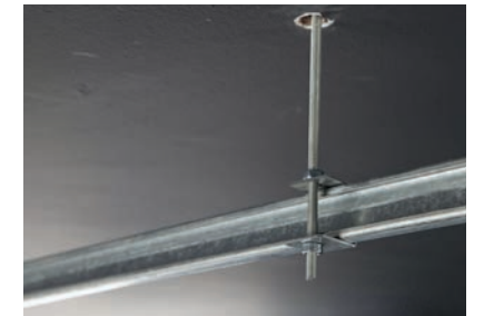
5. Join the suspension flange with the rod using the nuts.
