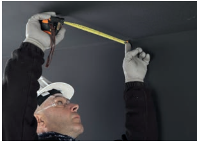
1. Lay out the location of the ceiling elements.
