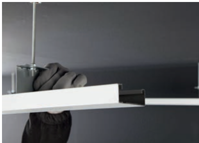
4. Install the hanging piece and the grooved profile.
