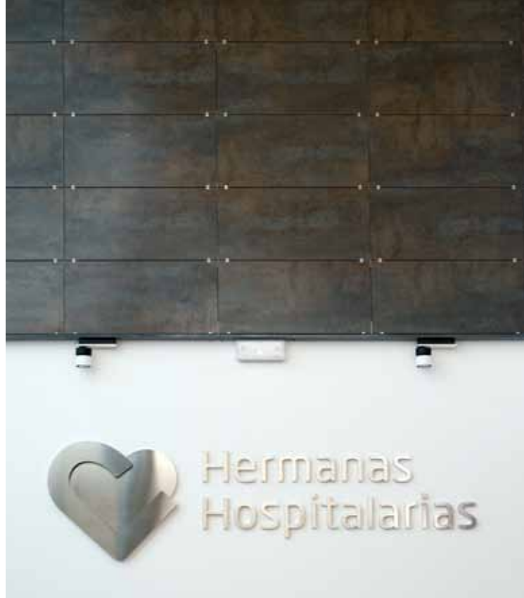
Cross-ventilated façade done in Ston-Ker ceramic (with a natural stone look that avoids the problems associated with this material) in two finishes: Sand Arizona , by Porcelanosa , and, for the connecting areas and the function room, Ferroker , by Venis , with a blued steel look (in 45 x 90 cm).
