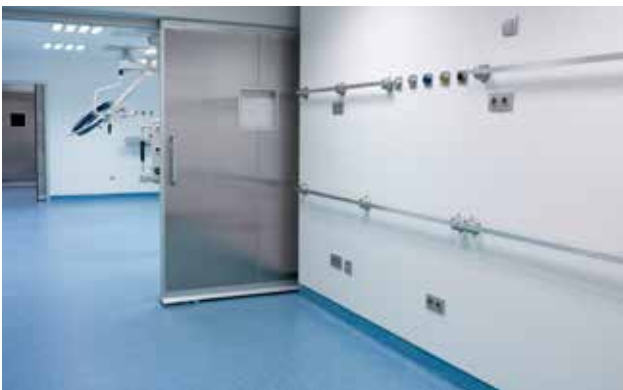
HOSPITAL PROVINCIAL (CASTELLÓN, SPAIN)
