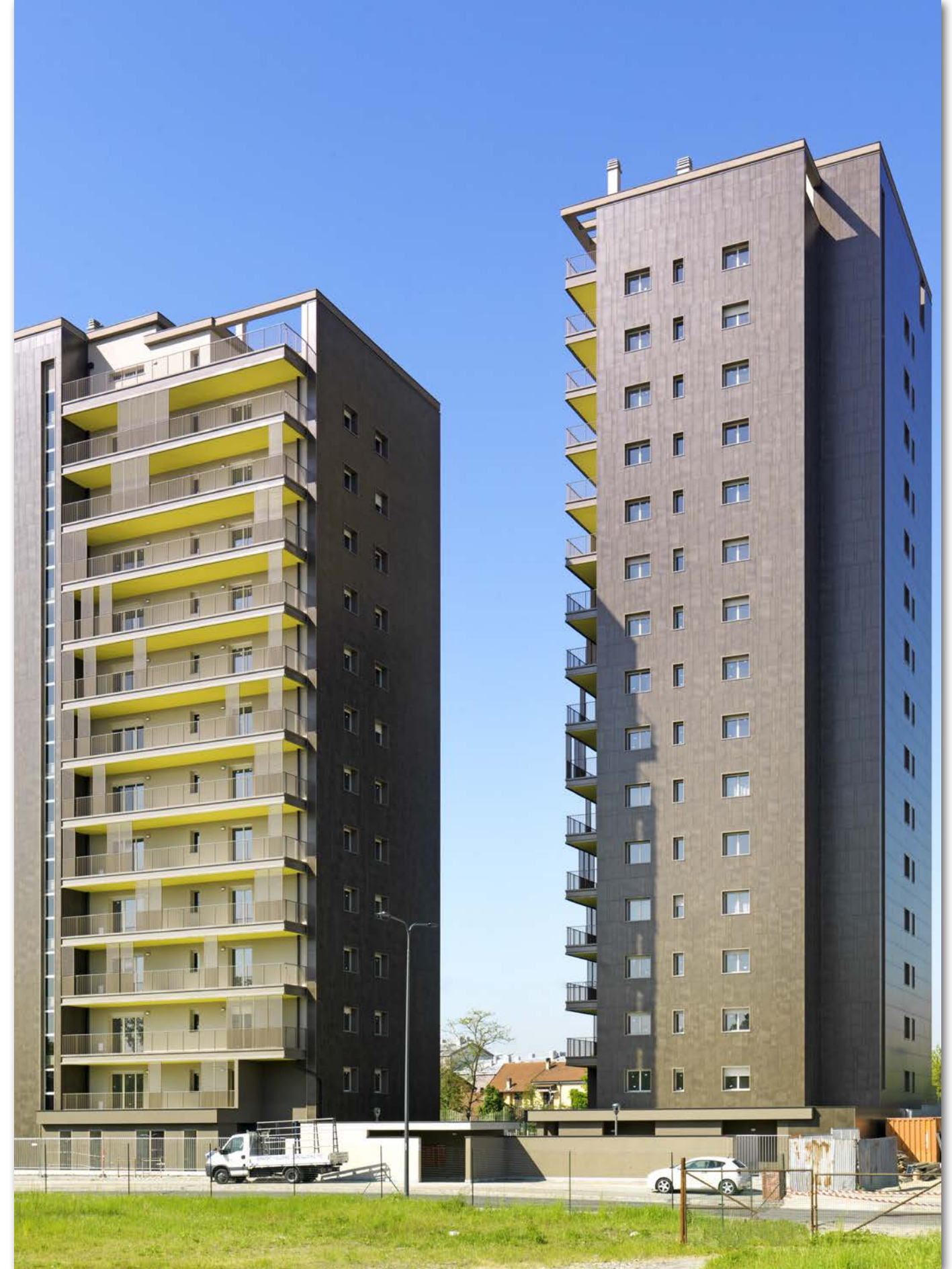
Via Castellmare, Milano, Italy
