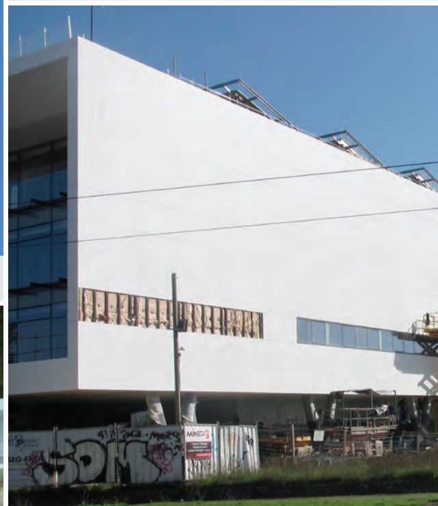
KRION® PANELS INSTALLATION
