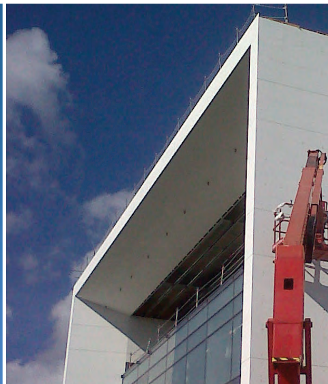
KRION® PANELS INSTALLATION
