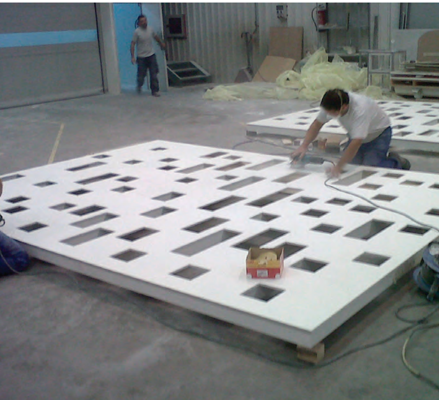
SANDING AND FINISHING OF PANELS
