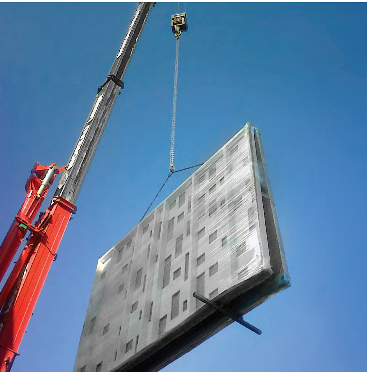
MOVEMENT OF PANELS IN SITE
