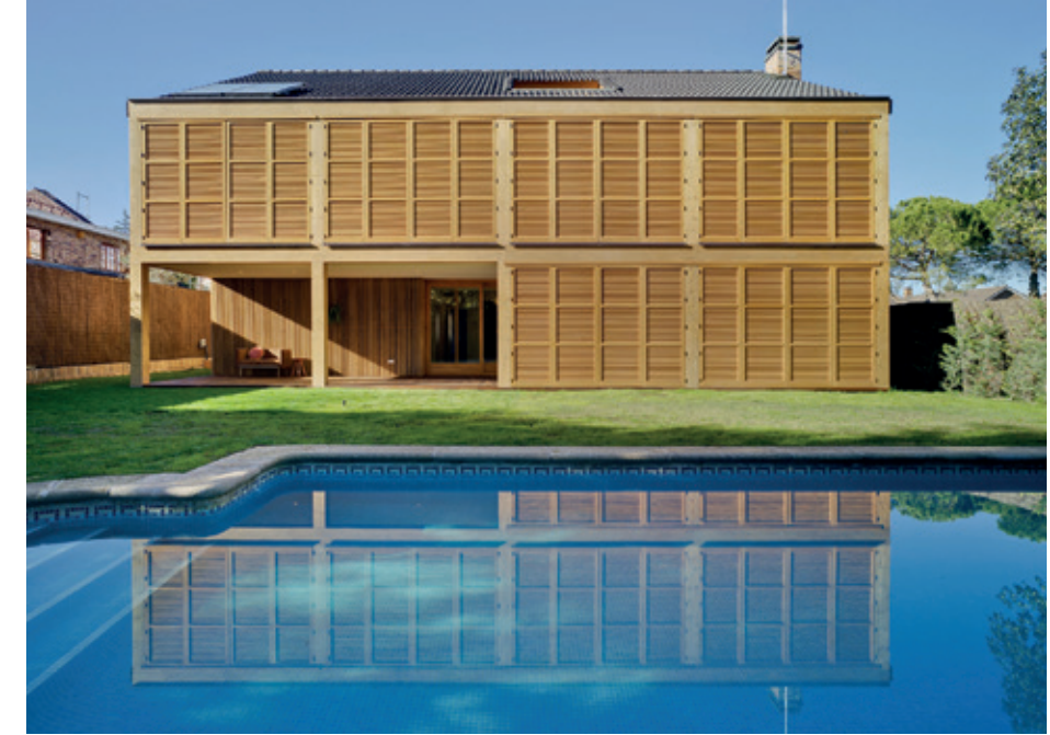
Much of this singular house by CSO Arquitectura and Commuty gives onto the garden, endowing it with a fresh and airy feel and allowing all the daylight in. Its Mallorcan shutters add an avant-garde eco-friendly appearance and architectural uniqueness.
