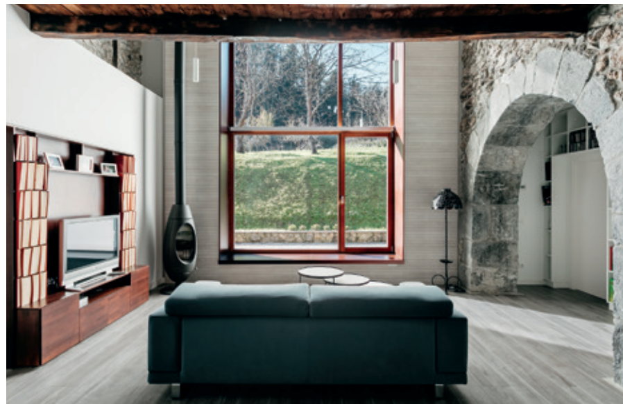
One of the most important changes was the modification of the house's original timber frame to connect the ground floor (the former stable) and the first floor, to create a double-height room. In the living room, PAR-KER® Steel Oxford wall cladding strips, 31.6 cm x 90 cm, by Porcelanosa were used. The floor was done in Hampton Grey, 22 cm x 90 cm, by Venis .
