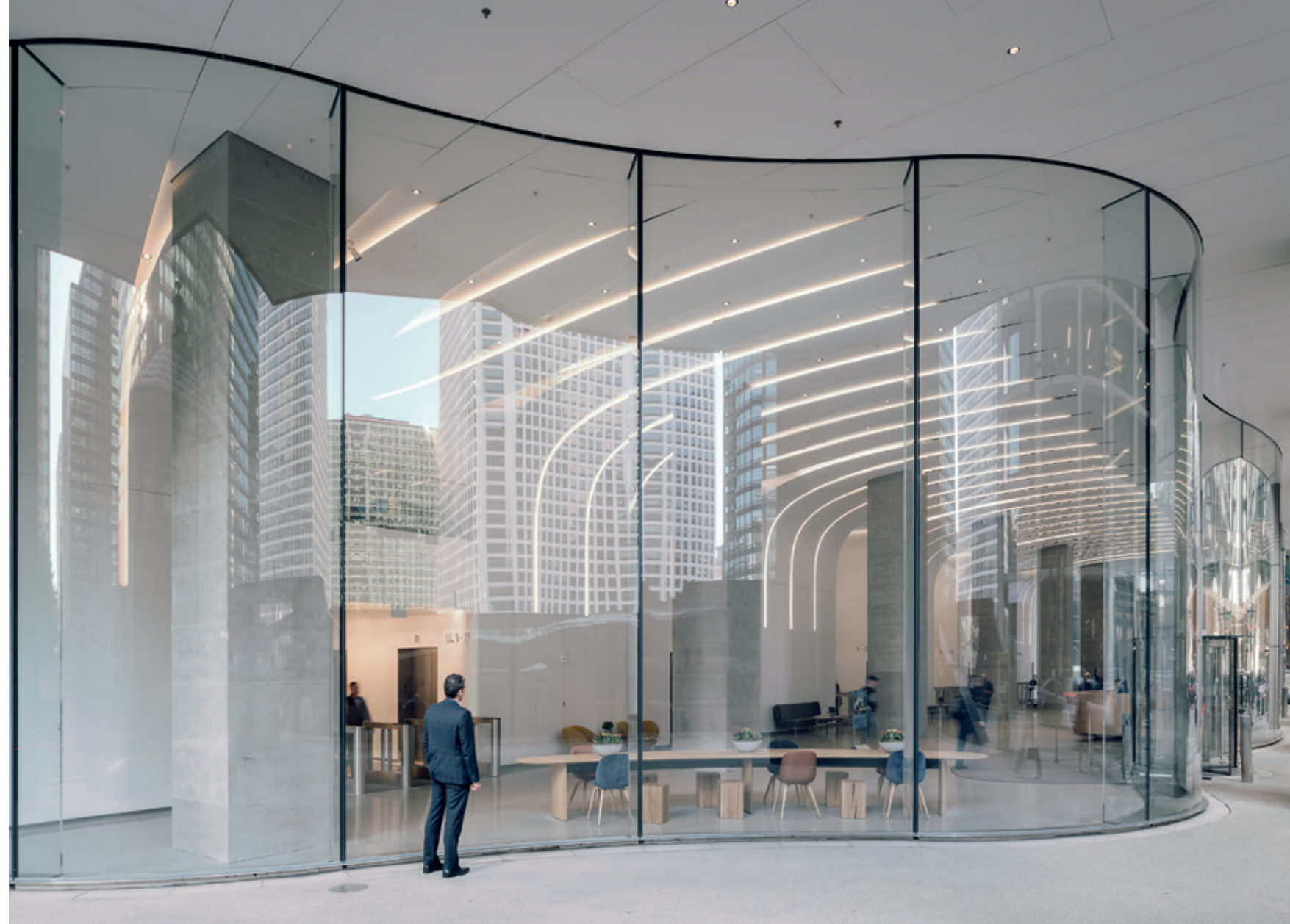
For the cladding and the ceiling, over 2,000 Krion® K-Life slabs were used which, in addition, support the curved glass panels of the new façade.
